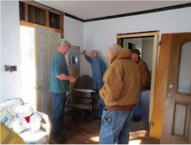
Randall Rosson checks the availability of circuits in the box after eliminating the need for electrical connections for the newer gas appliances. Photos by Judy
