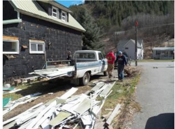
Kevin, Verne, and CJ start loading siding.
