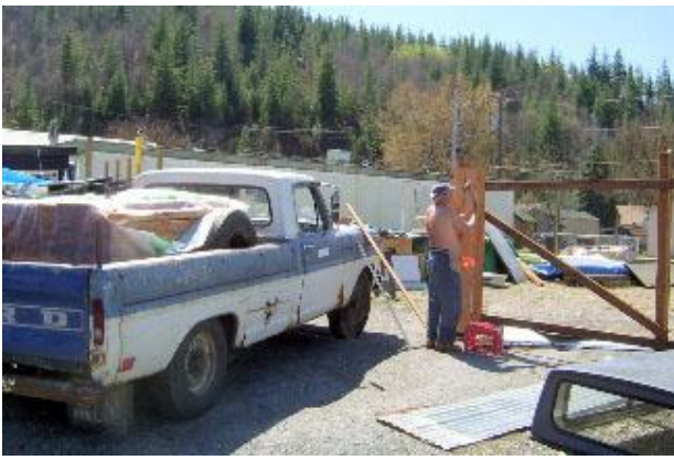
Verne starts nailing the cedar boards to the fence in back of the ReUse Store. He herded "Old Blue" carefully with 2400 lb of lumber on it. We need volunteers to help with projects like this outside as well as help in the store.
