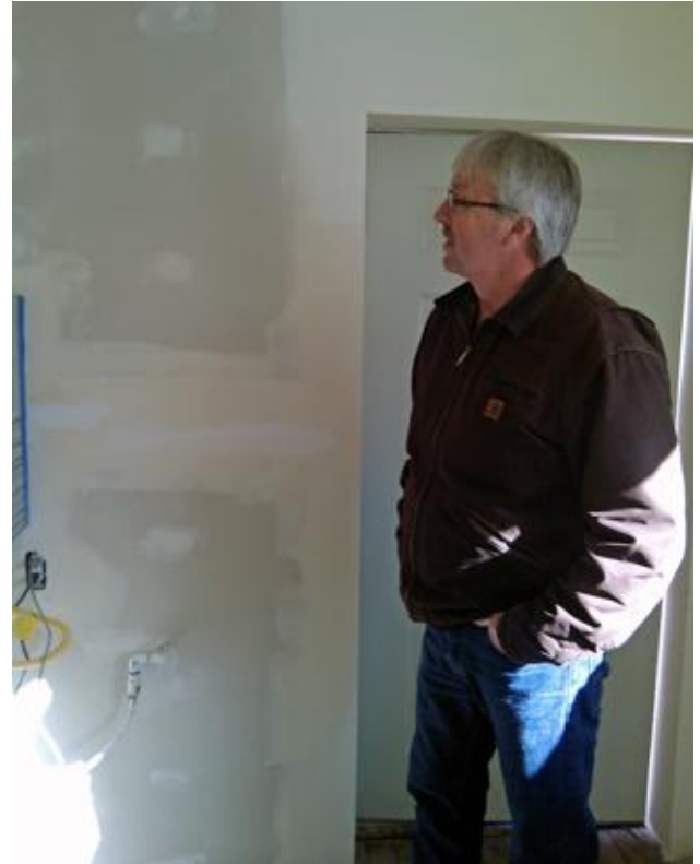
Shoshone County Building inspector, Mark Magnus, gives a final inspection of John Delaney's home before okaying his occupancy permit.
