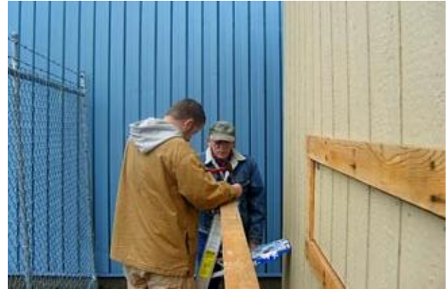
Chris & Bob work on the trim of the Little Shop Project
