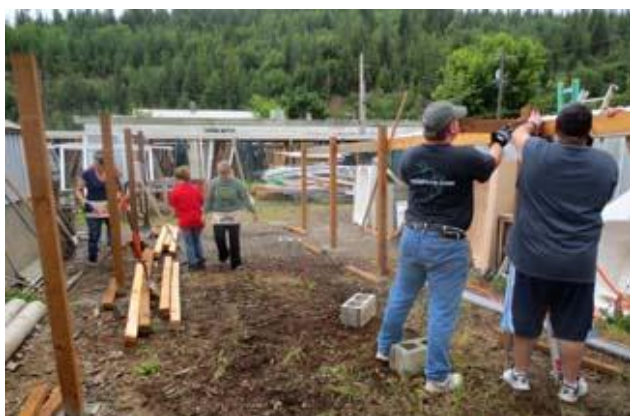
Part of the 2 nd week's crew of Idaho Servant Adventurer youth help Kevin & Mike Humphrey set posts in the back area to make more covered shelving.
