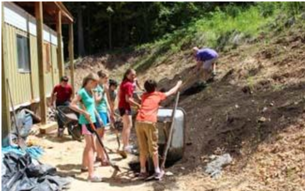
Boys ran the wheelbarrows full of soil and waiting shovelers tossed it up the slope. Others planted donated flowers such as iris and strawberries to hold the hillside in place.
