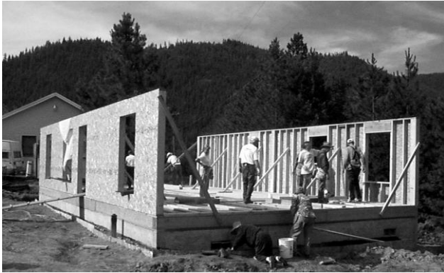
And the walls go up!
