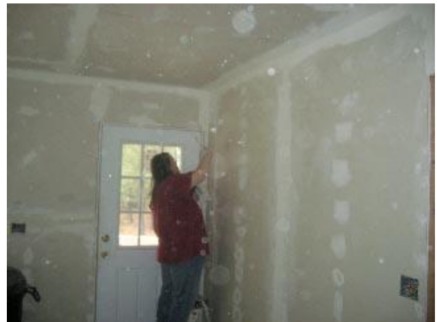
Darnell Kriedeman muds the wall by the front door at the Lake home.
