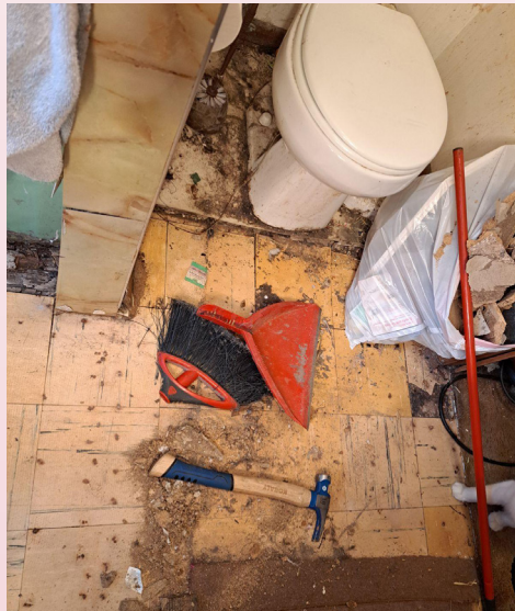
Photos of the damaged subfloors prior to Josh's repair efforts.
