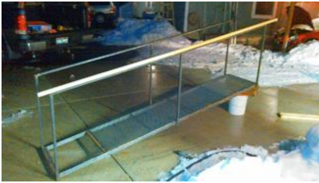
This ramp was designed by Bob Otto and members of The Friends of Nehemiah group of the Pinehurst Community Bible Church in Pinehurst. With its metal grid, there should be little snow shoveling. ☺ Photo by Bob Otto
