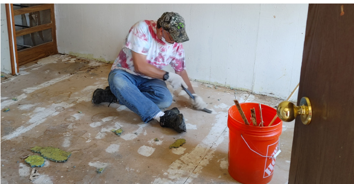
Brian Canterbury works on the floor.
