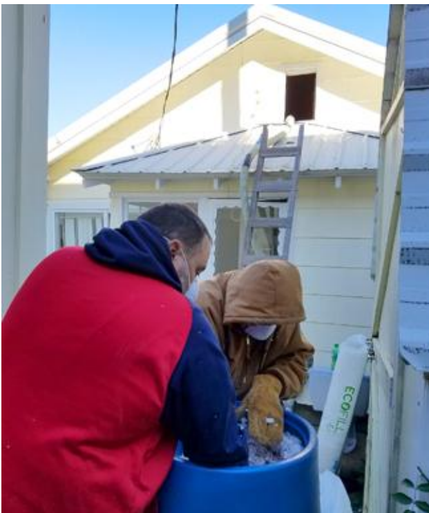
While John Boy Delaney directs the insulation inside the attic, Mike Humphrey and Verne Blalack stuff the bats of insulation into the blower.
