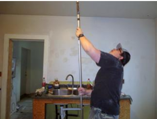
Nathaniel Galford puts the first coat on the kitchen ceiling.
