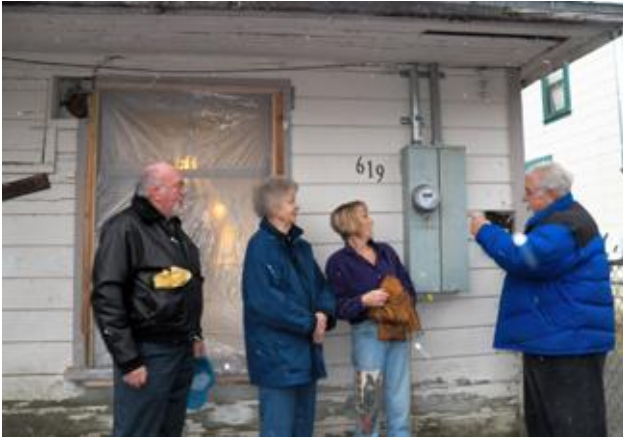
Rev. Phil Squire, R'Gean Lillibridge, Shannan Souza and Duane Little admire the repaired wiring which included replacement of old fuse boxes and duct tape splices on Shannan's home.
