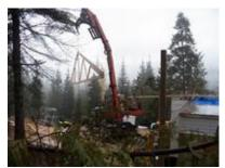
Dave Weingart uses his log loader to lift the trusses onto the roof.
