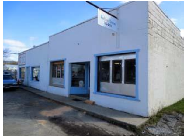
The ReUse Store is becoming “greener” with new smaller thermo-pane windows at the right front of the building.
