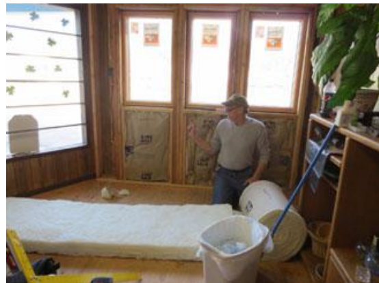
Joe Wolford cuts insulation to put around the new windows that replace a very large single pane window at the front of the store. Below he installs wallboard.
