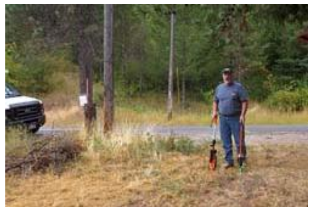
Joe Close from the South Fork Sewer District used a map and grid to locate the cleanout lid for the septic tank near the road. The Sewer District sends a truck every three months to pump out the holding tank since there is no adequate room for a drain field. It was important to locate the tank before heavy equipment moves in to set the new power-pole.
