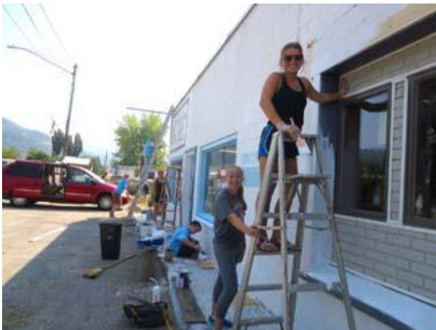
Our last youth group continues the painting the ReUse Store.
