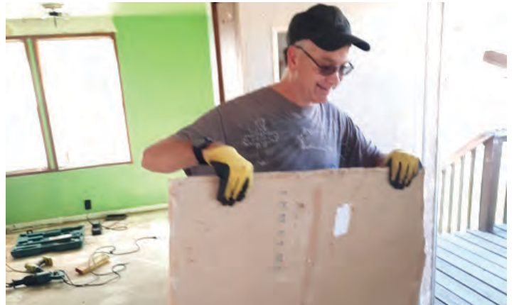
Brian Canterbury carries old sheetrock out of Brian's trailer.
