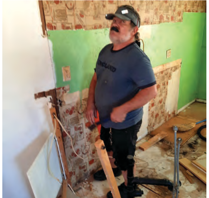
Don Mathews works on sheetrock.
