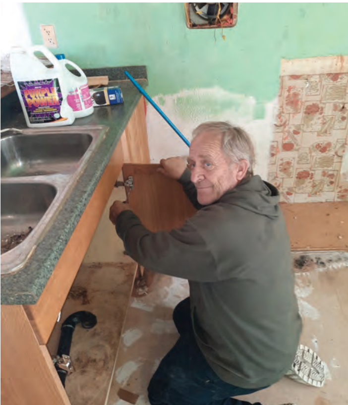
Ken Fairchild removes old kitchen cabinets.
