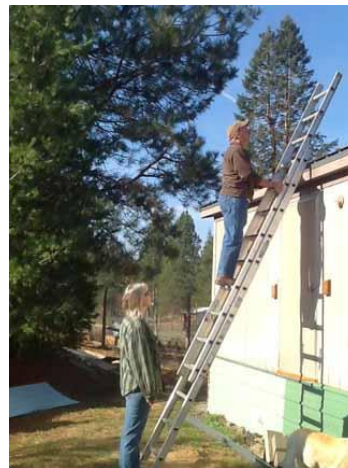
While Shannon Wood removes old shingles at right, Verne uses a flash light inside a vent hole to examine the framing of the manufactured home's roof. The rafters are very narrow, limiting the weight load. Photo by John "Boy"
