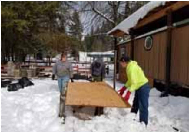
As Krista Kirby and John Boy Delaney hold them, John Hopper saws the skirting boards to fit the space below the trailer home.
