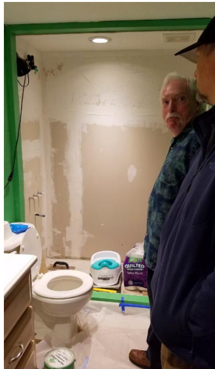
Barry listens to George explain how to fix the leaking pipe. Photo by Judy
