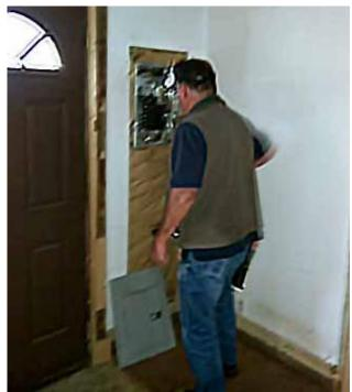
Electrical inspector, Don Geiger, checks the circuit box in the Osburn house. The main wiring passed inspection, but a new buried line has to be installed to the garage.
