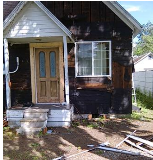
The youth have been stripping off the old siding, pulling out the nails and then stacking the wood for recycling after Verne sawed it up. This certainly has changed the appearance of the house and shows off the door donated by Shoshone Glass. John "Boy" stripped and finished it before Rick Gilbert reframed and installed it.
