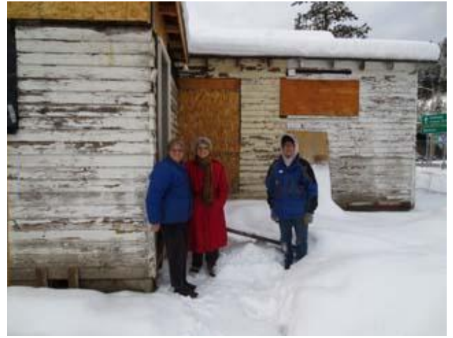
Ellie and Judy visit with John “Boy” at the Osburn house. Construction is halted until warmer weather. Photo by Kayla Blalack
