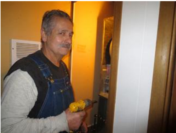
Jeff Crawford installs Melody's new furnace. Photo by Melody
