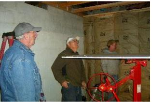
Using Jim Taylor's lift, volunteers, Norm Holtz and Rick Wood, help Verne (center) install a new ceiling in a small room at the ReUse Store. They will insulate it after the lights are lowered.
