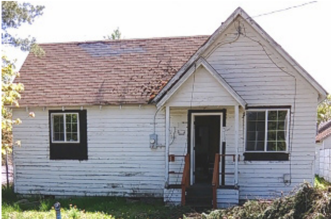
Front view of John Boy's house prior to beginning work
