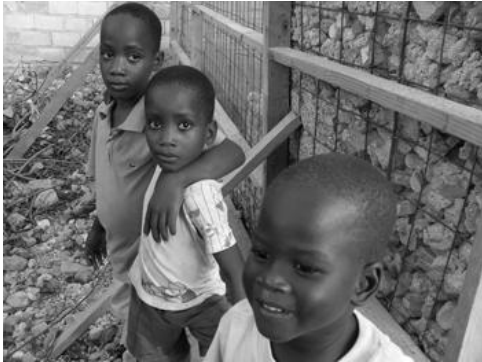
Children stand in front of a home being built with recycled earthquake rubble.
