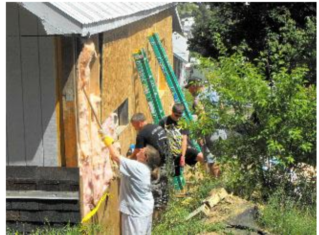
The youth install insulation in the new outer wall.
