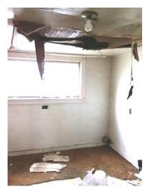
This house in Osburn will require significant work on the rear of the house where water has leaked through the ceiling. If we buy it, this could be a good project for the 2 Fuller Center Bicyclist groups when they stay to work.
